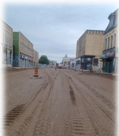
Talbot Street graded with granular 'B' ready for subdrains and curb
